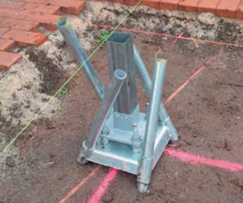
S250 with fully adjustable stump assembly - Domestic Project
