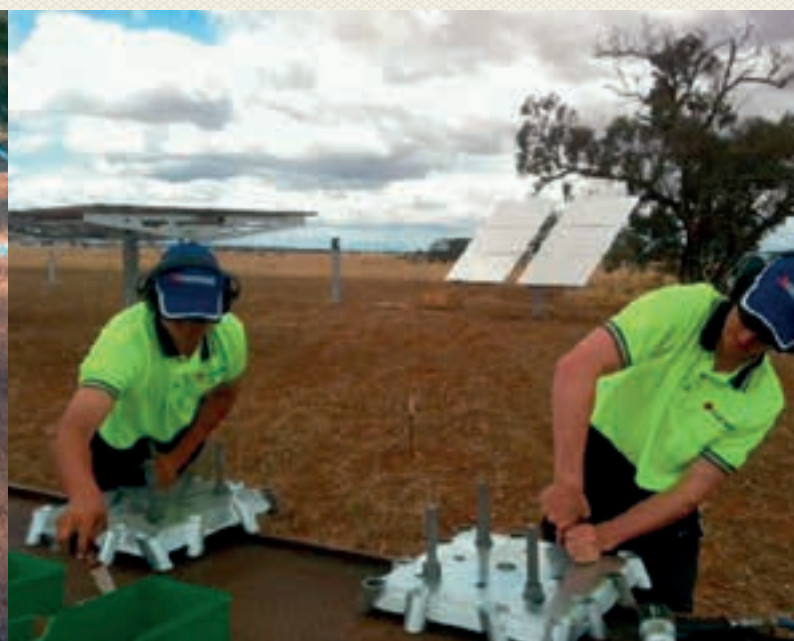
Assembly of nuts and bolts
