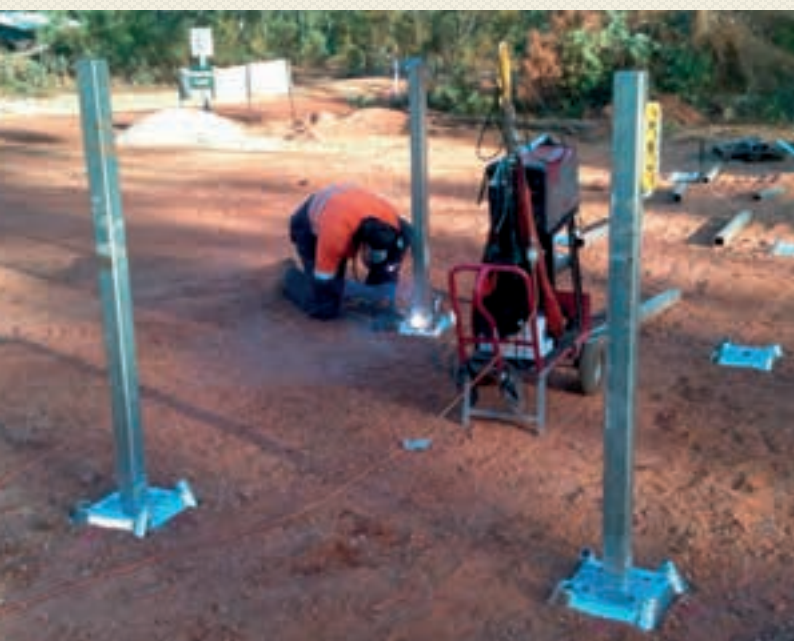
Welding directly to Surefoot
